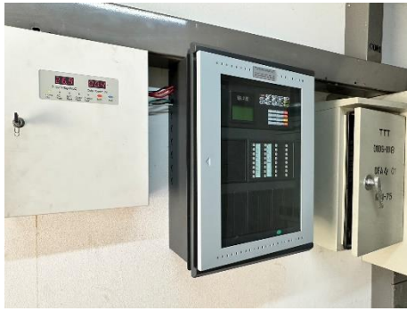
Fire Alarm Control Panel: FCP
